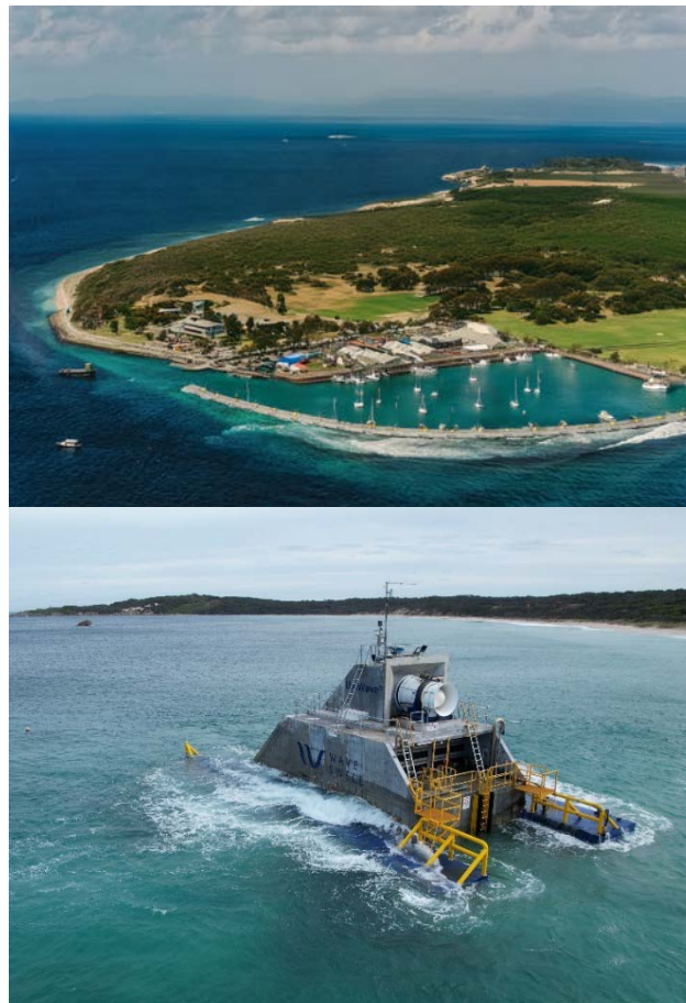
Figure 5. (Top) Conceptual example of Wave Swell Energy's device as a CSI-WEC. (Bottom) Wave Swell Energy's UniWave200 WEC deployed at King Island, Tasmania.
