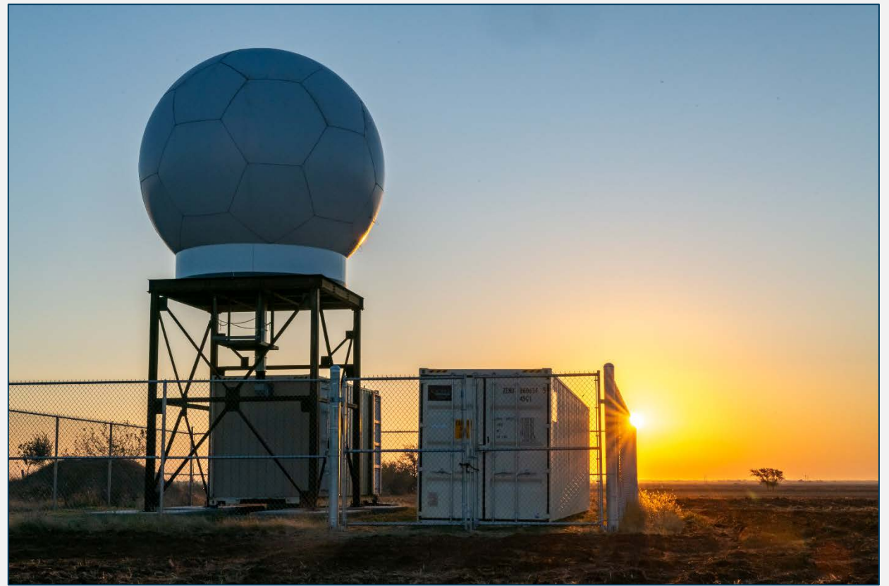
X-Band Radar Measurement installation near the King Plains Wind Farm, Garber, Oklahoma. Courtesy of Bryan Bechtold / NREL
