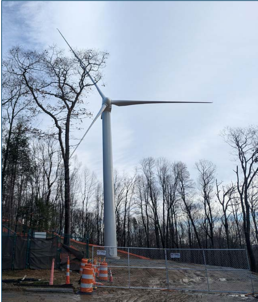
A poorly sited DW system. Courtesy of Brent Summerville.
