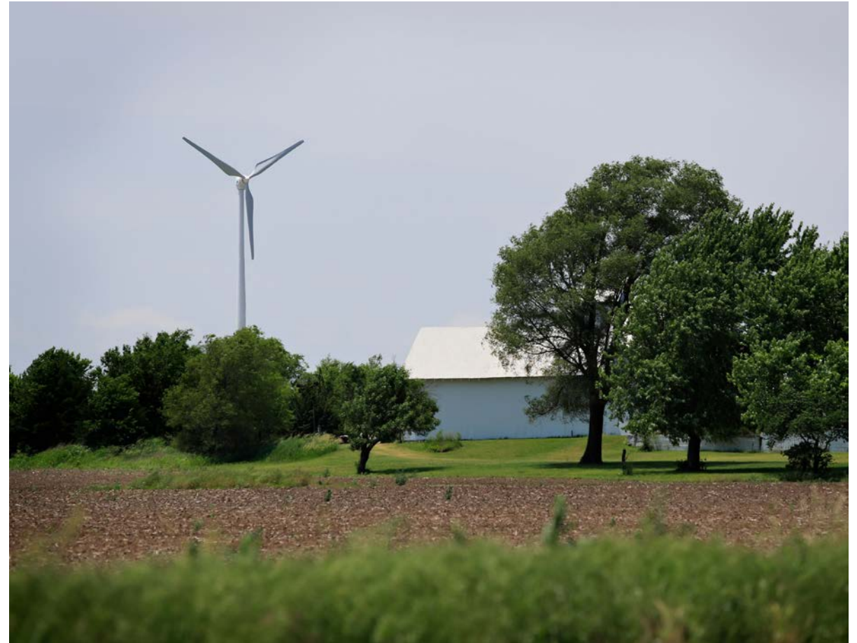
Eocycle S-16 installed in Kansas. Photo from Eocycle America
