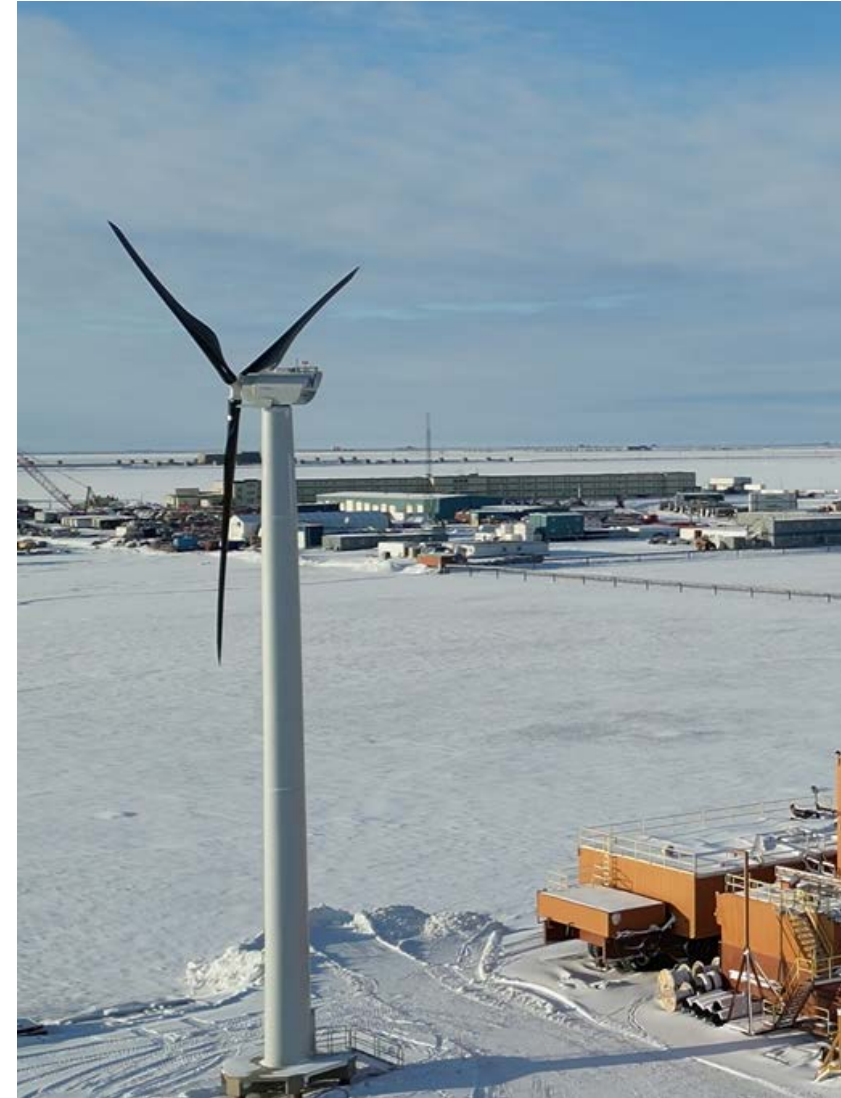
Northern Power Systems returns to the U.S. in 2023 with this Prudhoe Bay installation. Photo from Chris Connor, NPS
