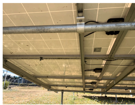
Fig. 4. Rear side photo of modules was taken from the site located in Portland. The surface of the backsheet has been contaminated by biological materials.
