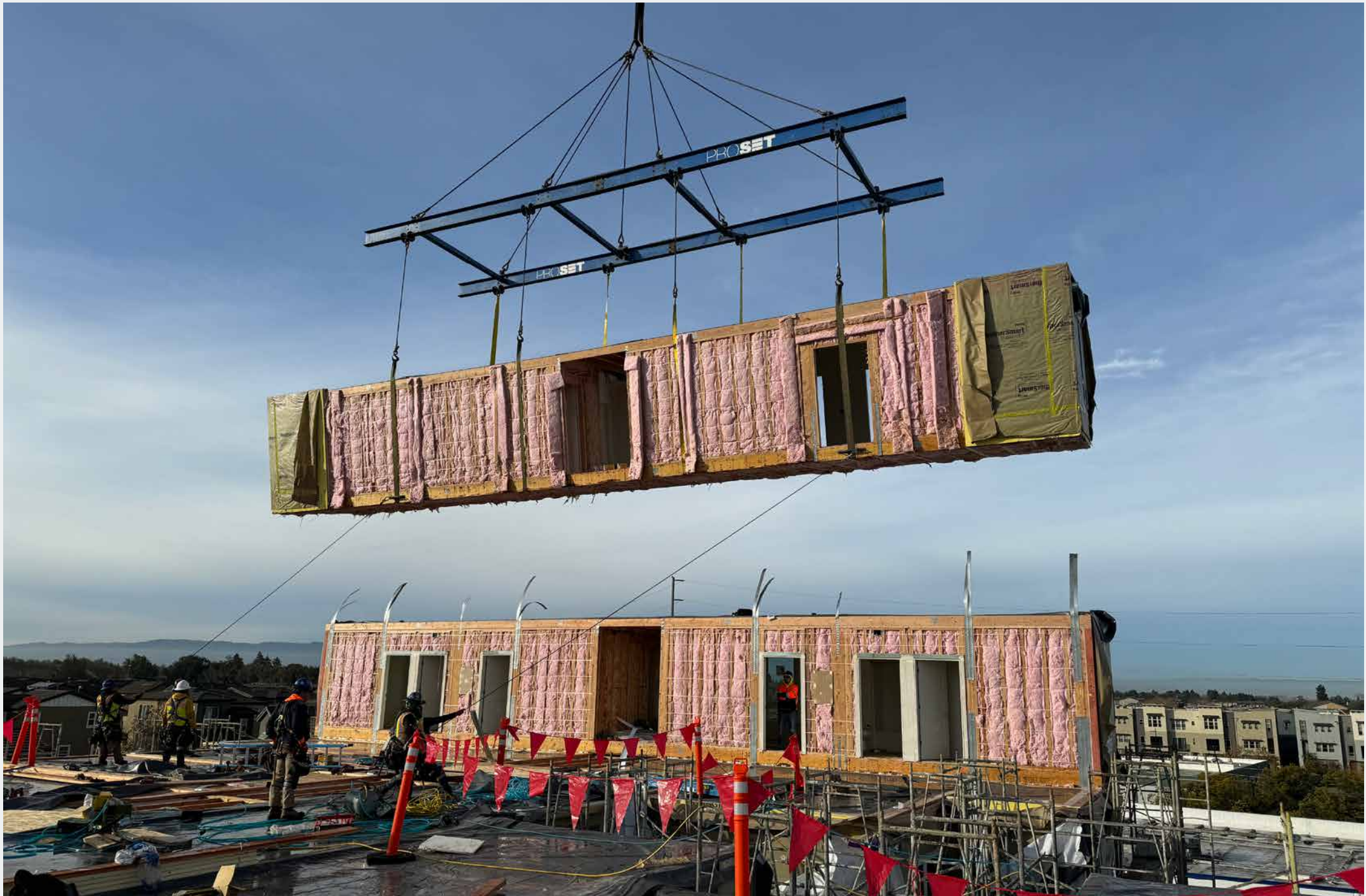
Figure 23. A set crew guides and positions a modular unit Photo from ProSet LLC
