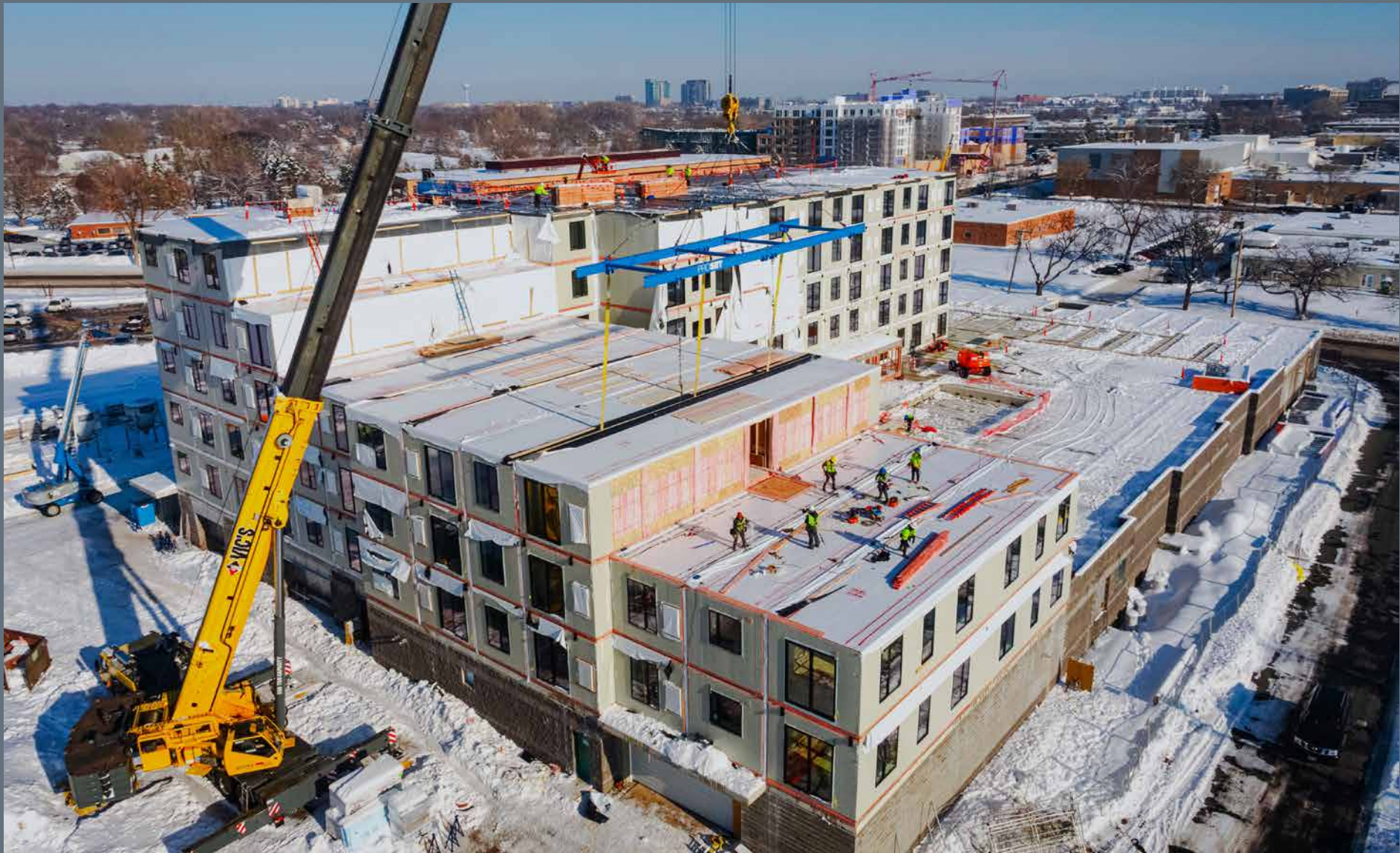
Figure 14. Proset LLC’s landing team guides a modular unit into place and prepares to tie the unit in
