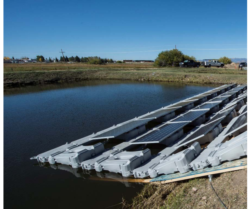
Photo by Dennis Schroeder, NREL 53264
