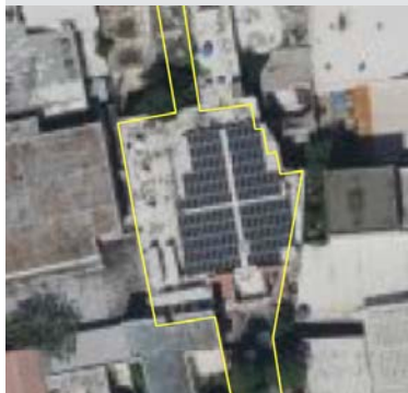
Existing rooftop PV observed on Fox Former Delicias Theater/Mall (Brownfields), Ponce
