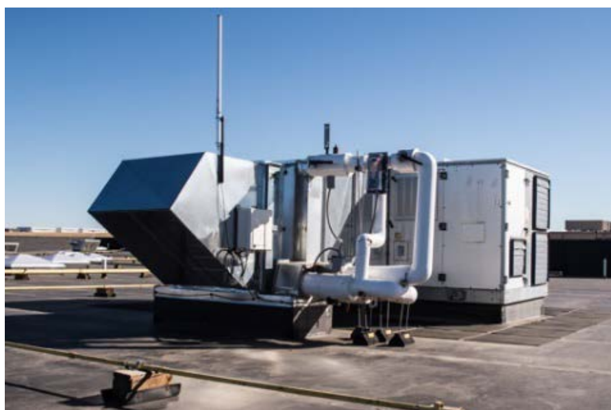
Figure 11. Example of buildings in the Rooftop Units, Non-Food Service segment
