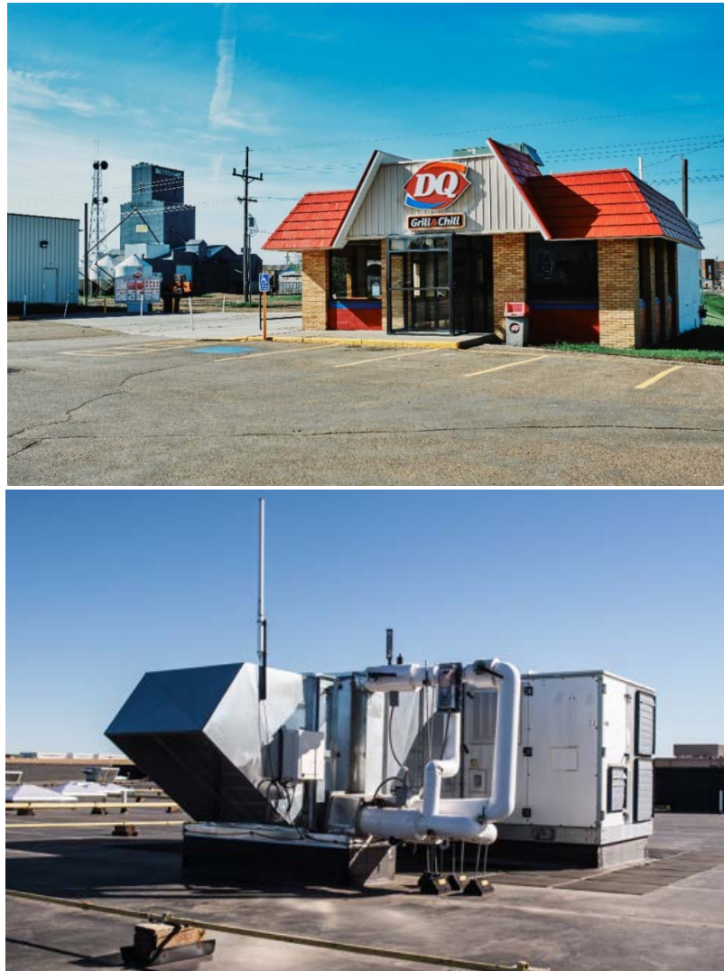
Figure 12. Example of buildings in the Rooftop Units, Food Service segment
