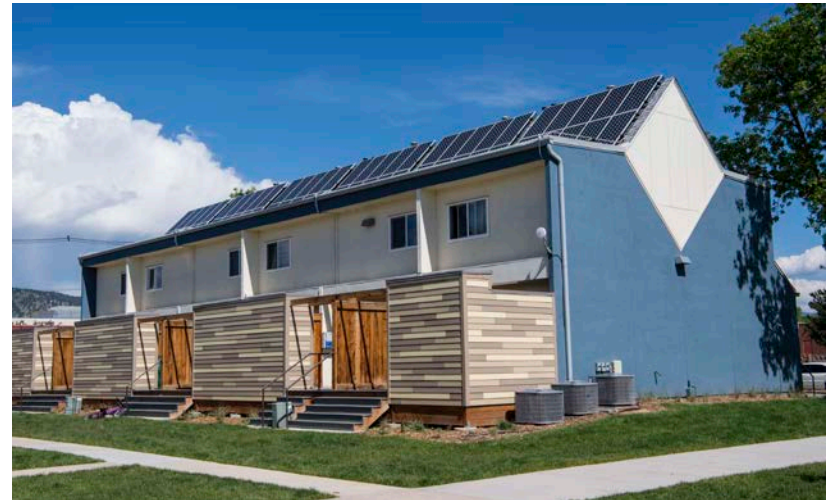
(Photo by Dennis Schroeder / NREL)
