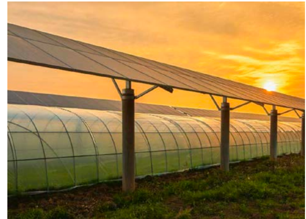
Solar PV panels on a greenhouse. Photo from iStock 1129147050
